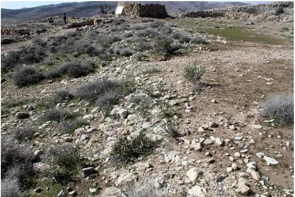
Fig. 7. Remains of a foundation (Photo by H. Abbasnia)
