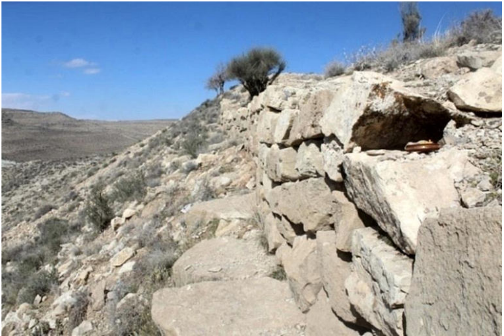
Fig. 10. Exterior fortification and the foundation (Photo by H. Abbasnia)
