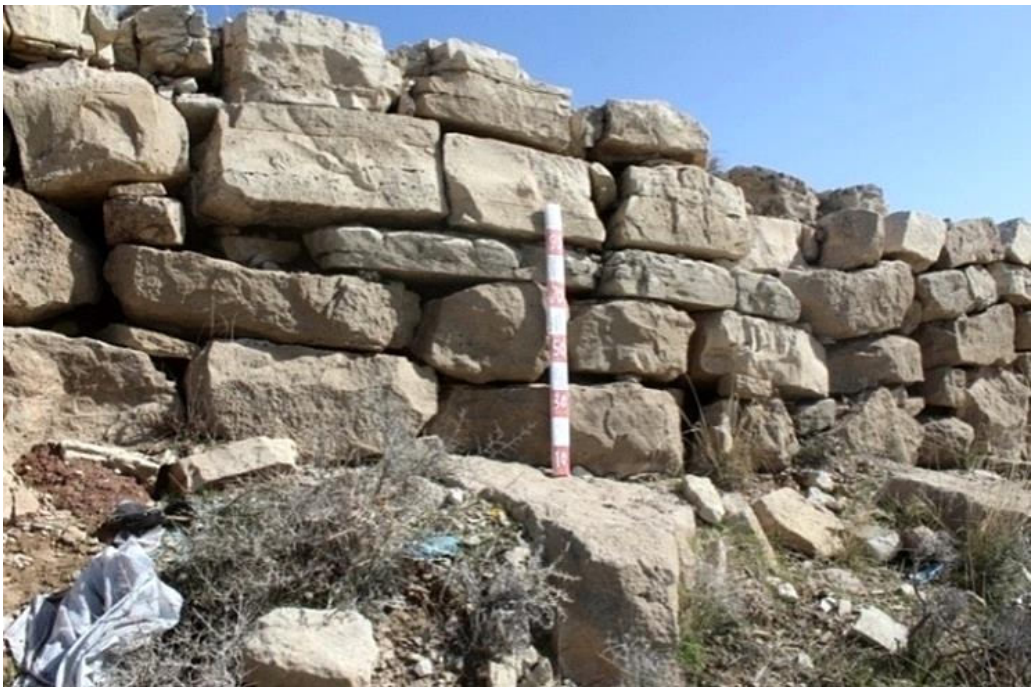
Fig. 9. Exterior fortification and the foundation (Photo by H. Abbasnia)
